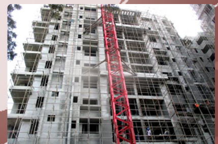
Tower E North side
