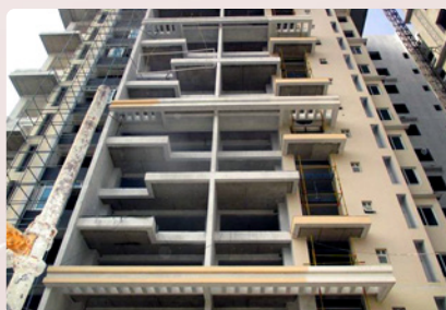
Tower A South side
